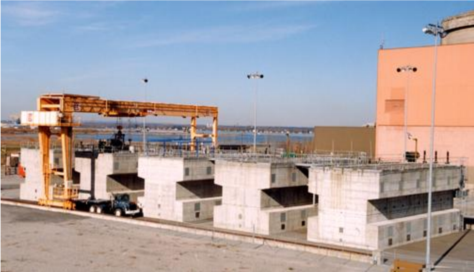
Photo from Hydro-Québec
