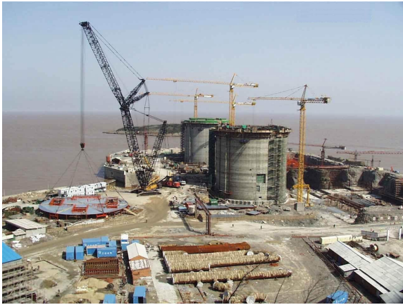
March 1999 – VHL – Temporary Roof
