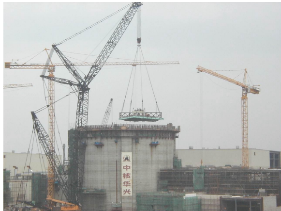
November 2000 – Dousing Module Lift
