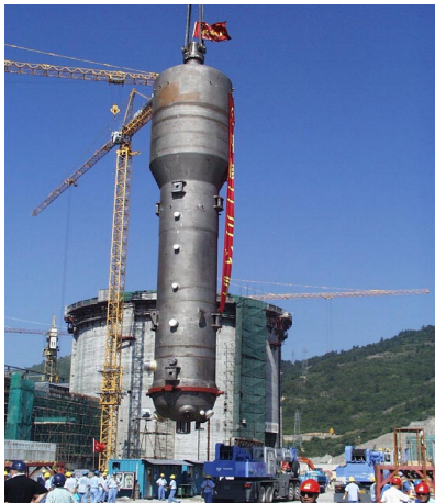
July 2000 - U1 Steam Generator Installation
