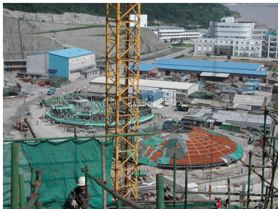
April 2001 – Temporary Roof
