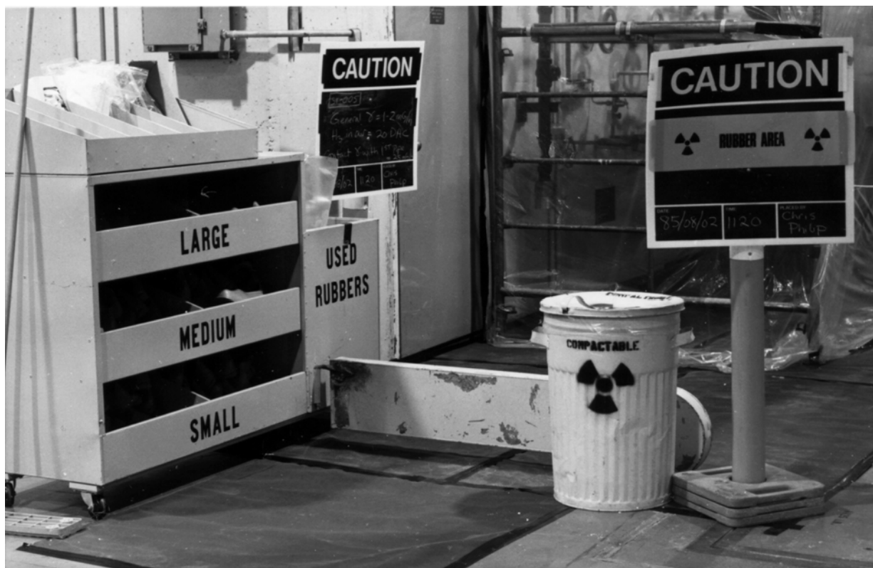
Fig. 9.17. Rubber Station at Entrance to Rubber Area
