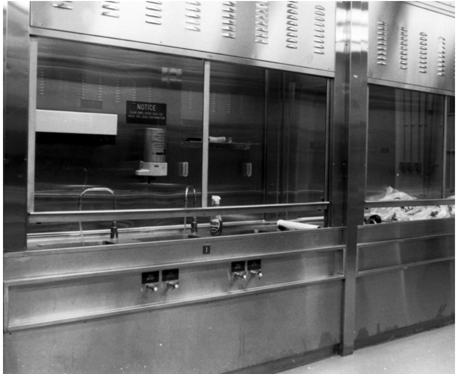
Fig. 9.22. Fume Hoods in the Decontamination Centre
